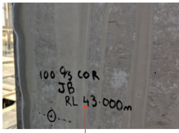
Example of RL mark by the Builder's Surveyor
