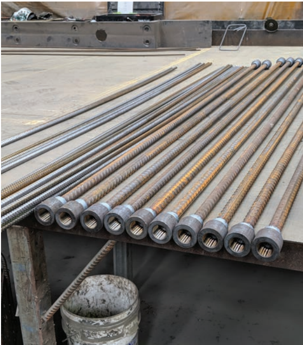
Reinforcement components on the cage fabrication bench
